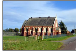
St Michael's Springbank Road, Springbank
