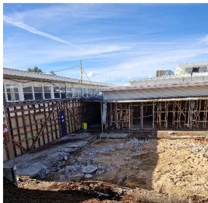
Demolition this week at St. Mary's
